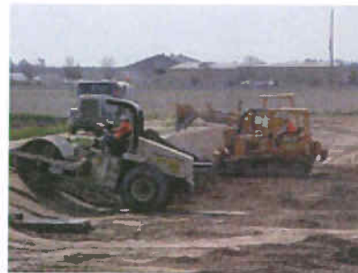
Compaction of soil-cement as a liner.
