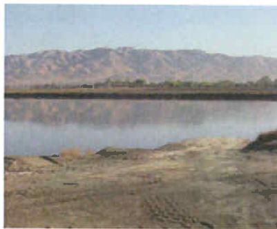
Flooded soil-cement lined drying bed.
