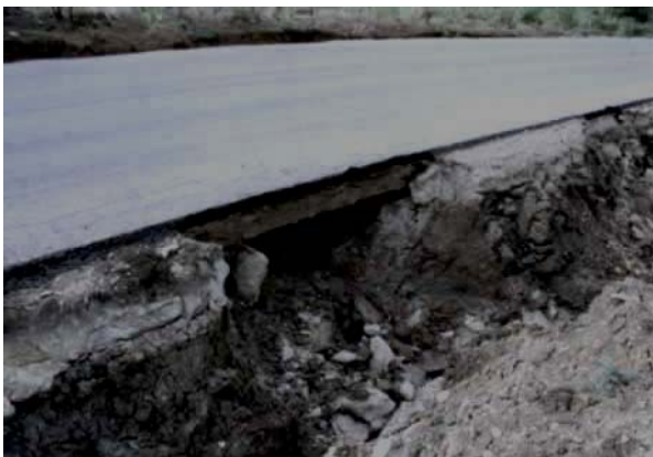
Stable Chemically Treated Base Undermined by Erosion
